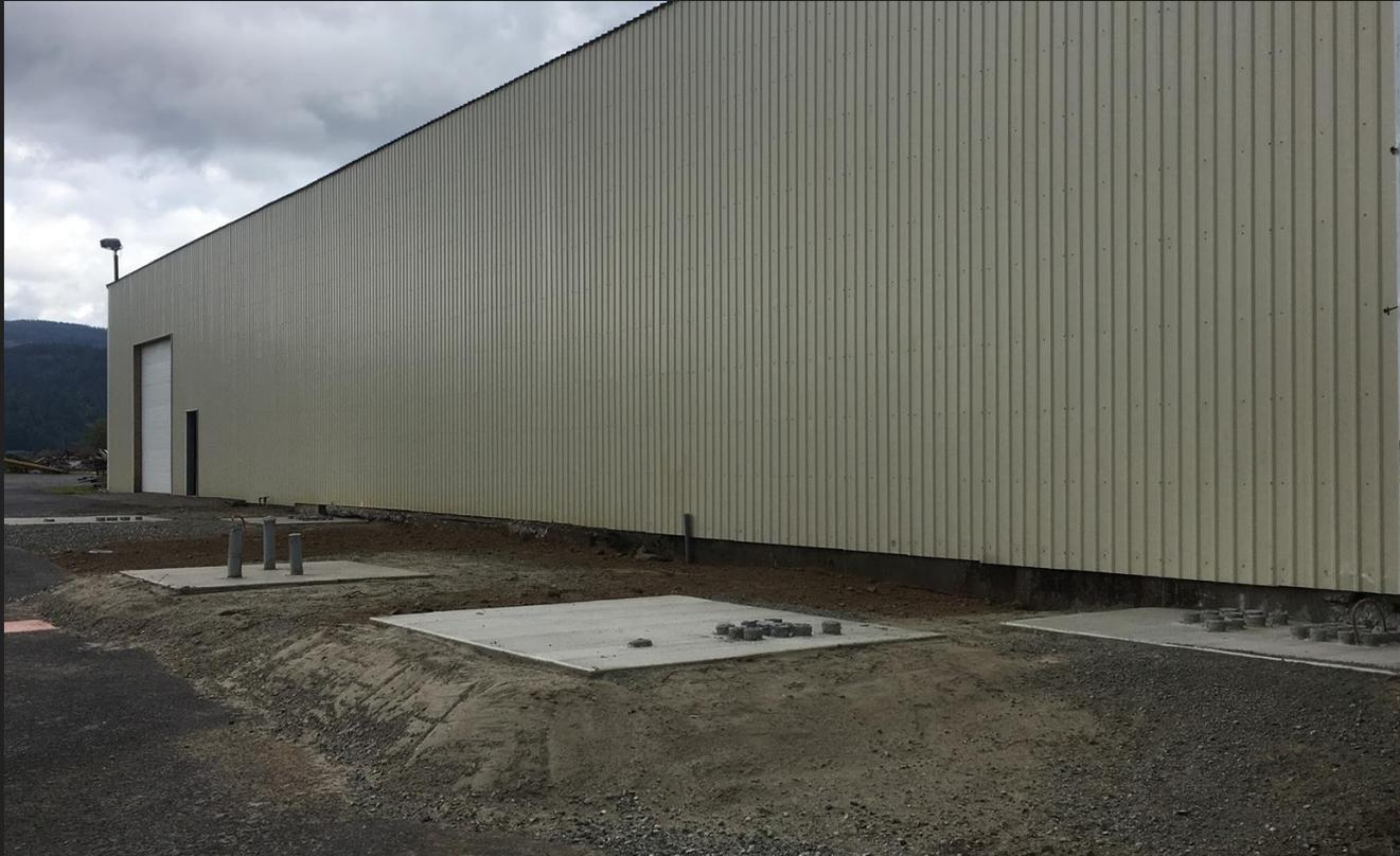
Soon this side of the building will be large intake fascia flanked by large transformers and switchgear. Fiber conduits were also laid.
